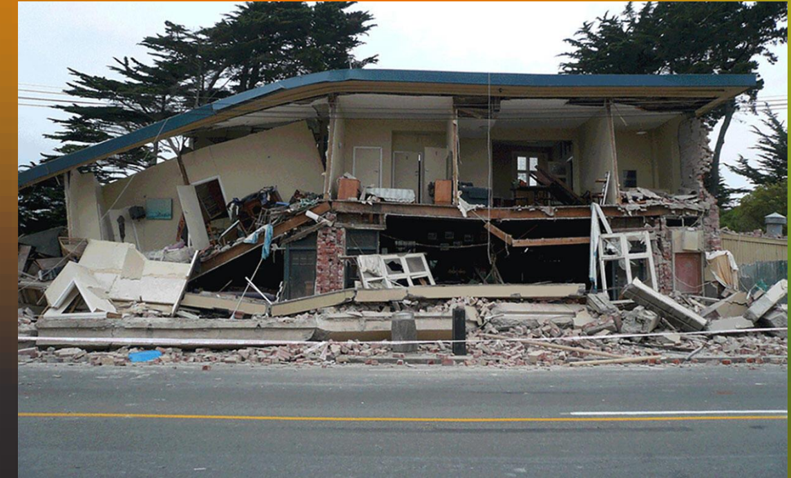
Building damaged by the February 2011 earthquake in Christchurch, New Zealand [ https://www.usgs.gov/media/images/earthquake-damaged-building-damaged-building ]
