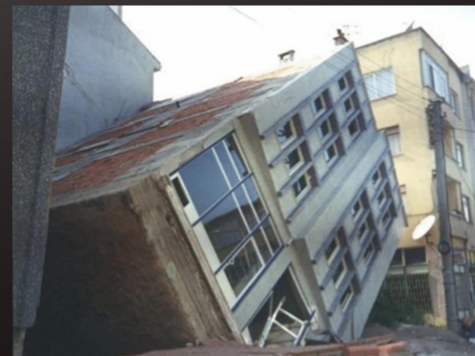
Example of an overall rotation of the base of the structure with an overturning motion during 1999 Kocaeli earthquake, Turkey [Bozzoni, F. et al., Bull. Earthq. Eng. 2021, 19, 4719–4744]
